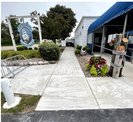
New Concrete along West Side of Building
